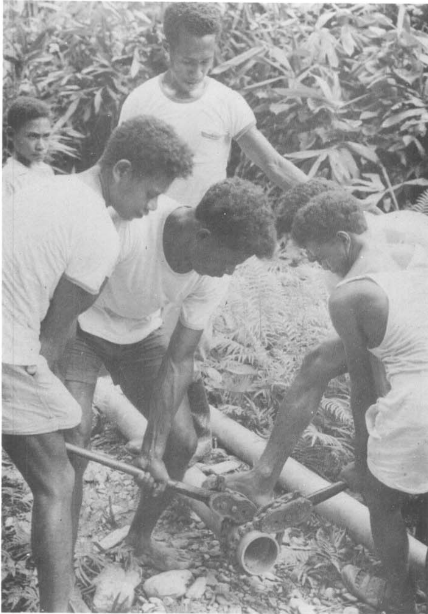
Water main being assembled.
