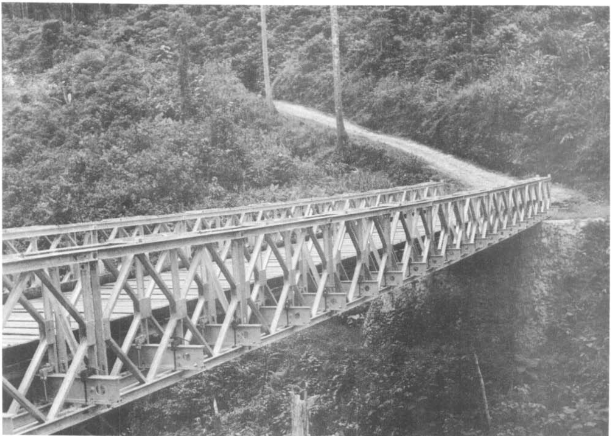
Bailey bridge carrying the Teminaboean-Ajamaroe road.
